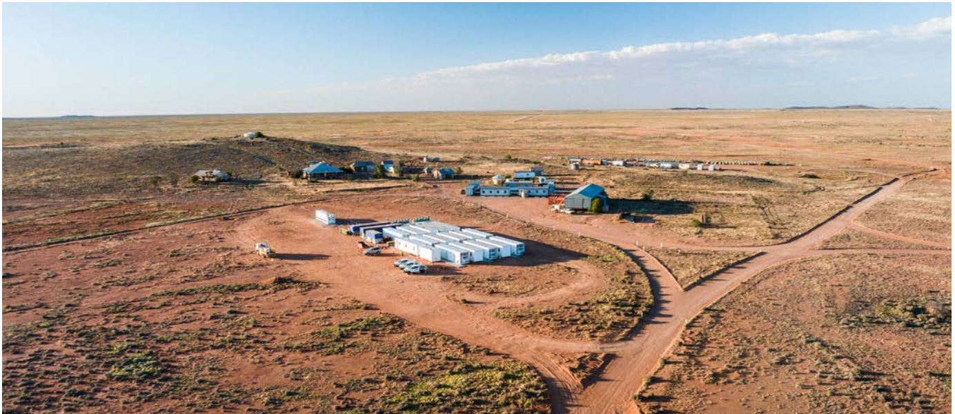
Figure 3 General view of the Kalkaroo homestead, camp and core yard, June 2023.
